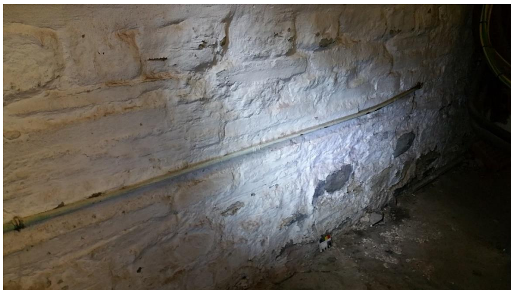
Wall construction in Area B (location 18)
