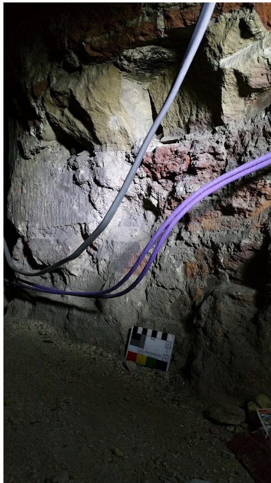
Wall break-through to crawlway (Location 39)
