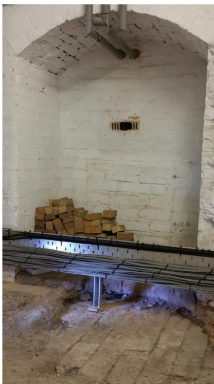
Fireplace or furnace alcove? (Location 33)
