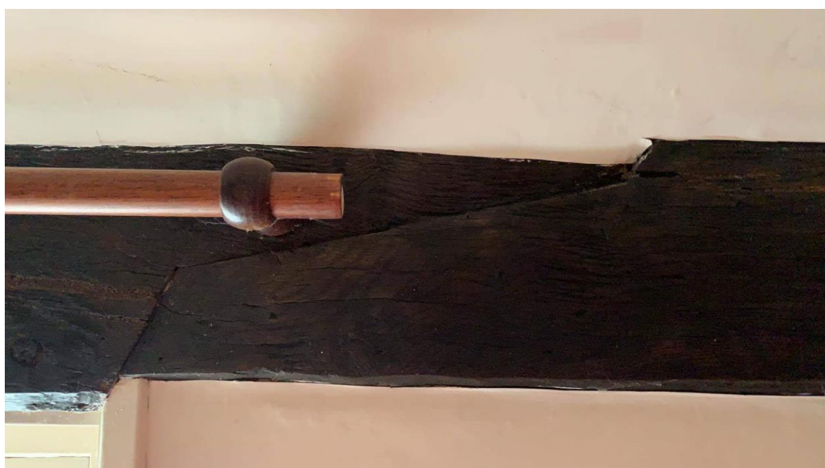
Figure 13 Joint of eastern wall plate, looking east (Photograph: Julia Parry-Jones)
