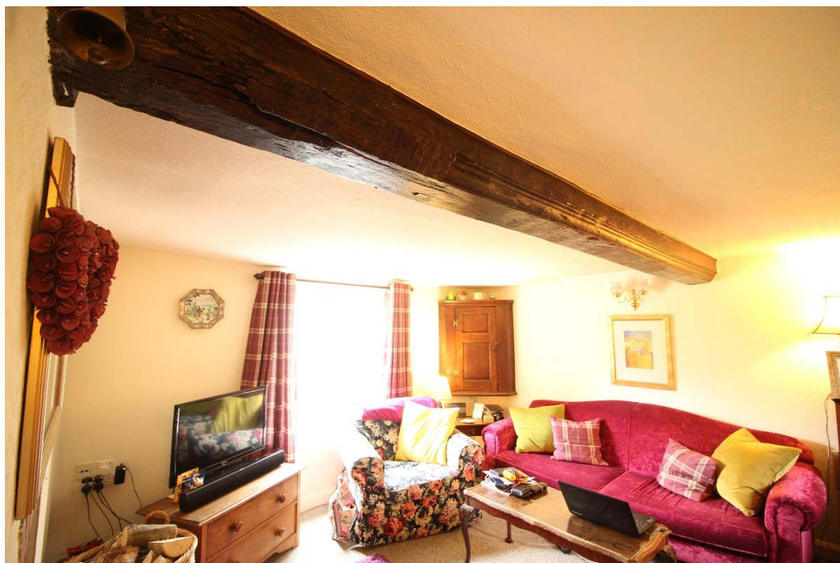
Figure 12 Spine beam of the ground floor south bay, note the moulding, looking south-east
