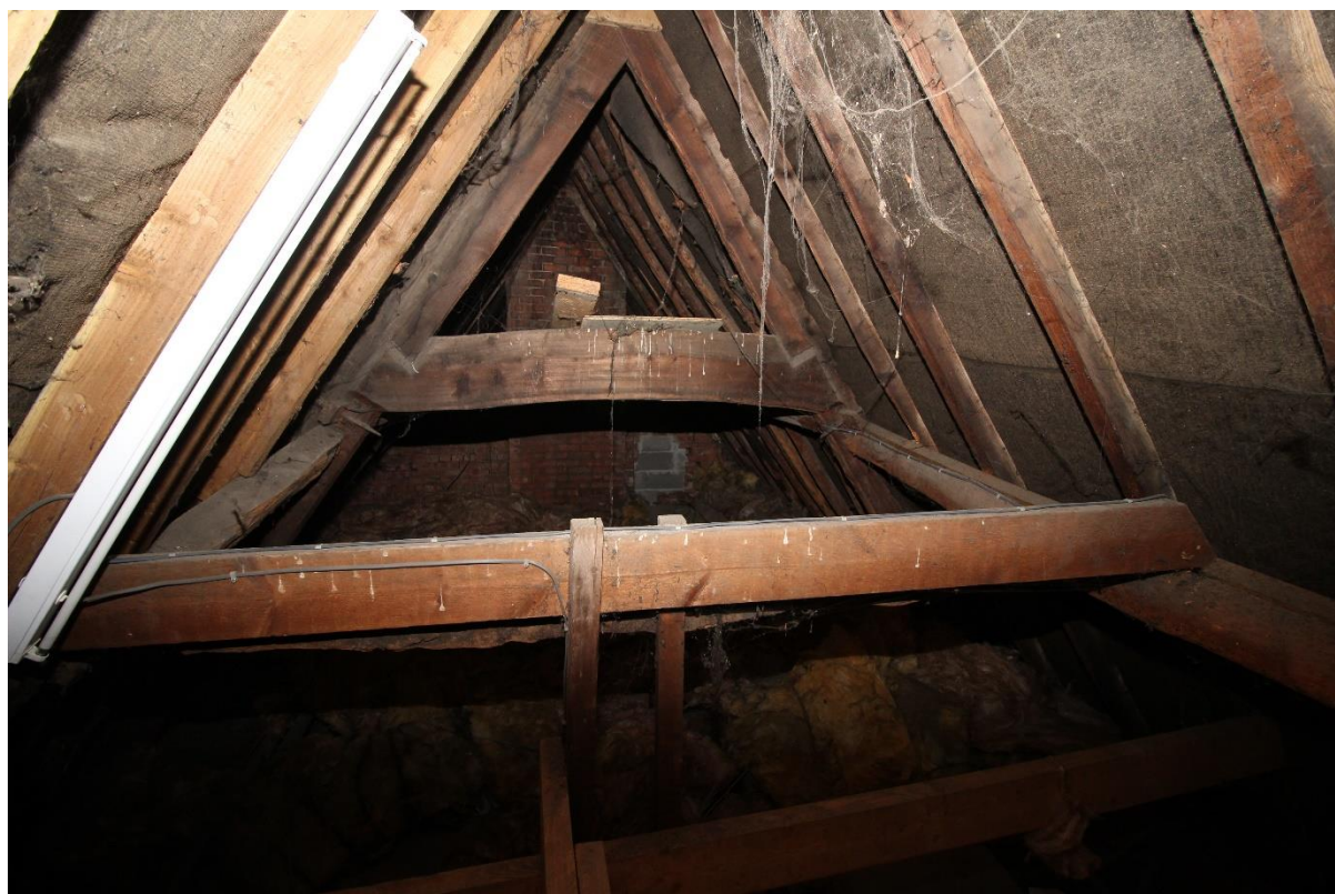
Figure 7 Softwood roof structure of the north-south range, looking south
