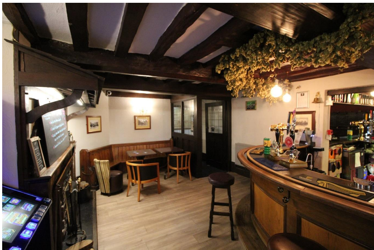
Figure 4 Main bar-room, looking north, note the chamfered bridging beam
