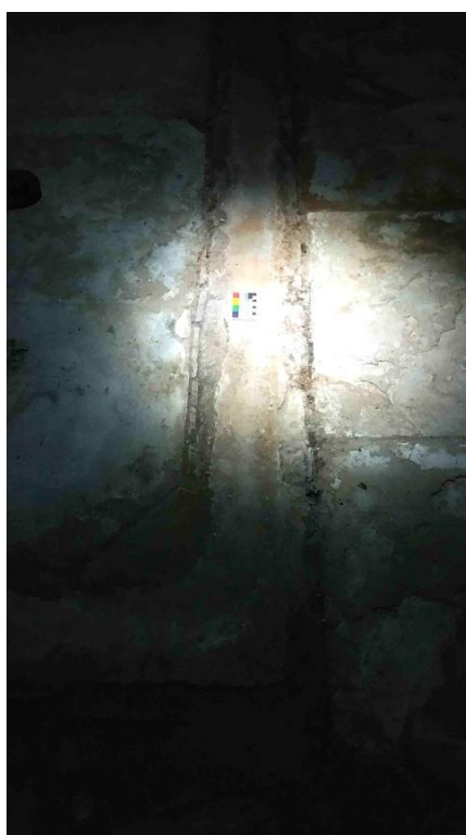
Characteristic stone slab floors with stone lined drainage channels in Area A (Location 8)
