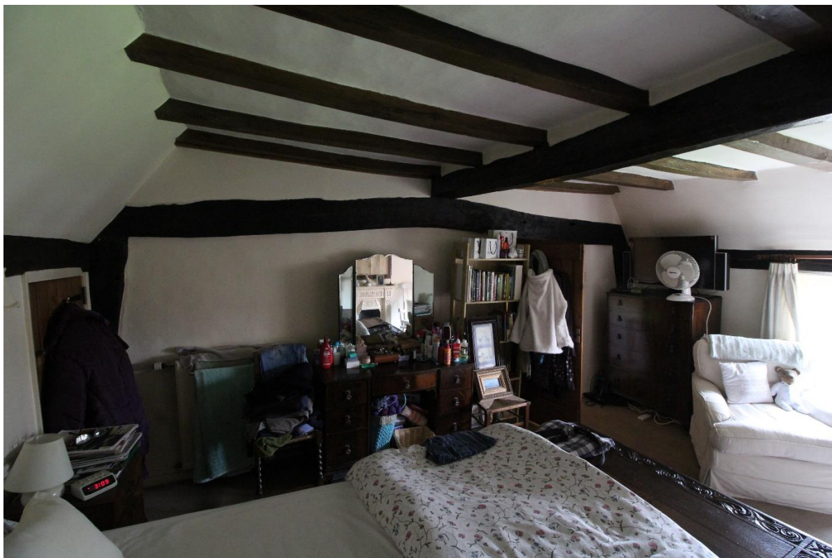
Figure 14 First floor central bay, note the cranked tie beam, looking north-east
