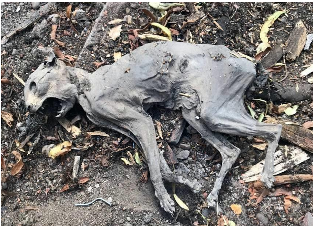
Figure 9 Ritually concealed cat discovered in the roof structure of the outshot over the cellar, looking east. (Photograph: Jonathan Pass)
