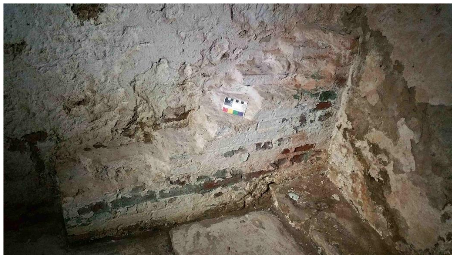
Construction in NW corner of room B15 – built using medieval brick.
