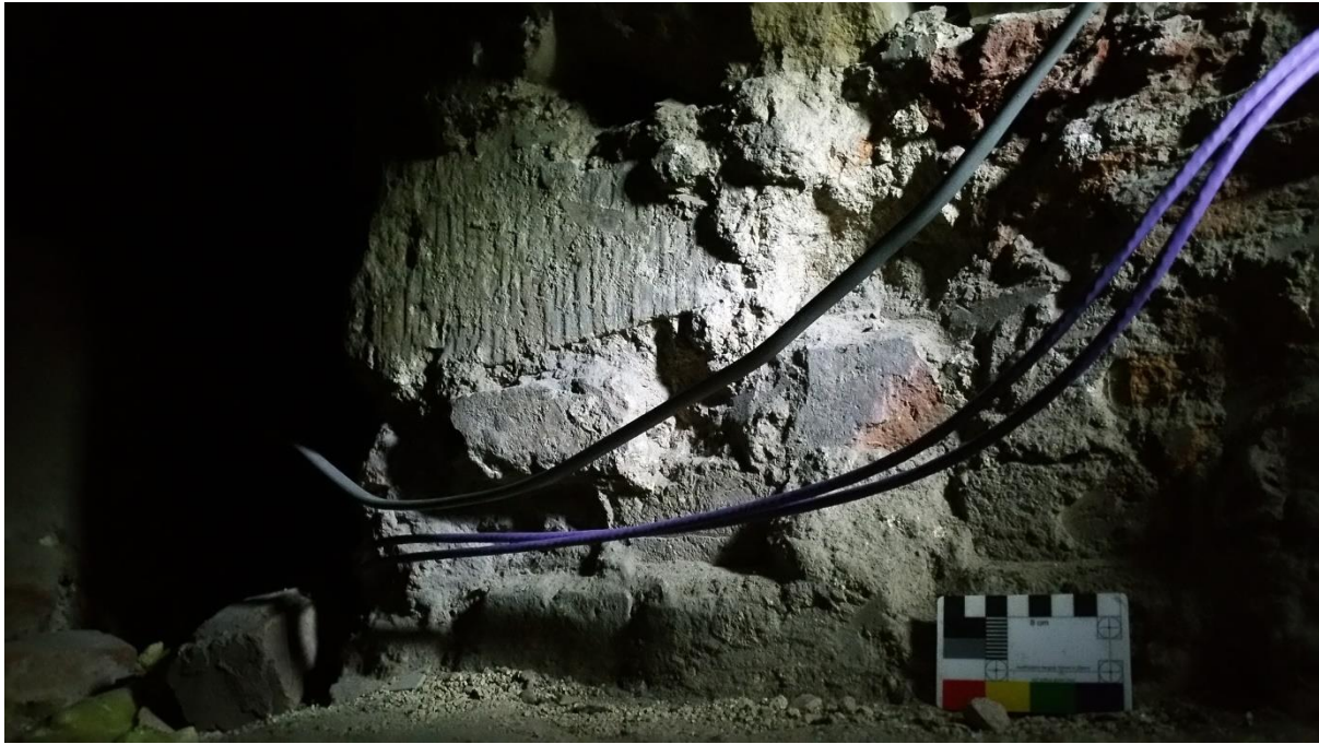
Wall break-through to crawlway (Location 39)
