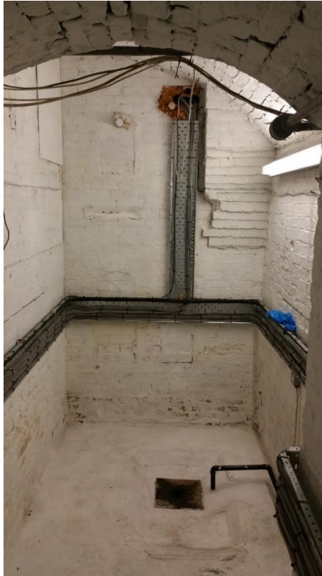
Boiler room? (Location 35)
