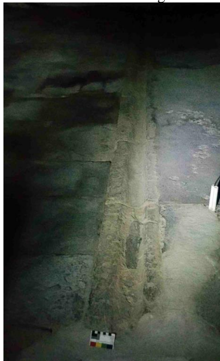
Stone lined drainage channels in flagstone floor
