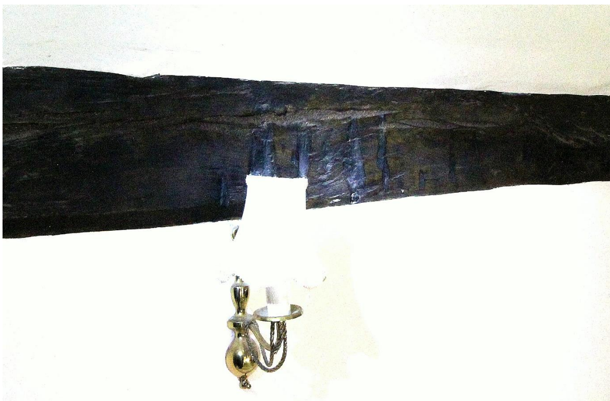
Figure 15 Ritual taper burn marks on the western wall plate of the central bay, note the centre-line drying crack in the timber, looking north-west
