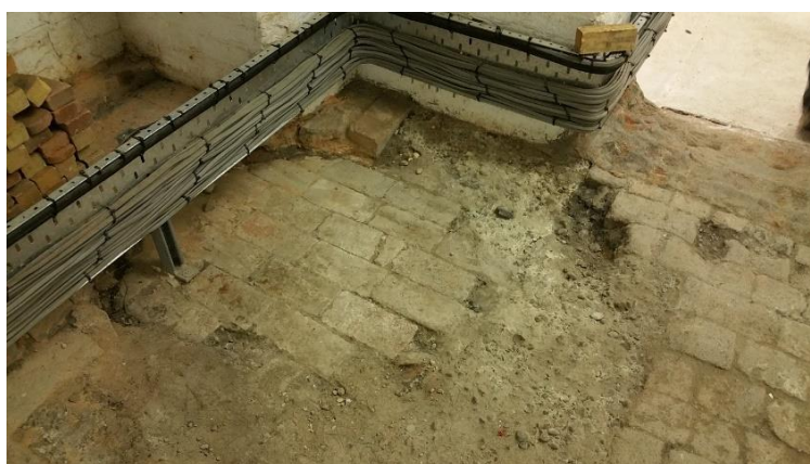
Circular feature in corridor (Location 34)
