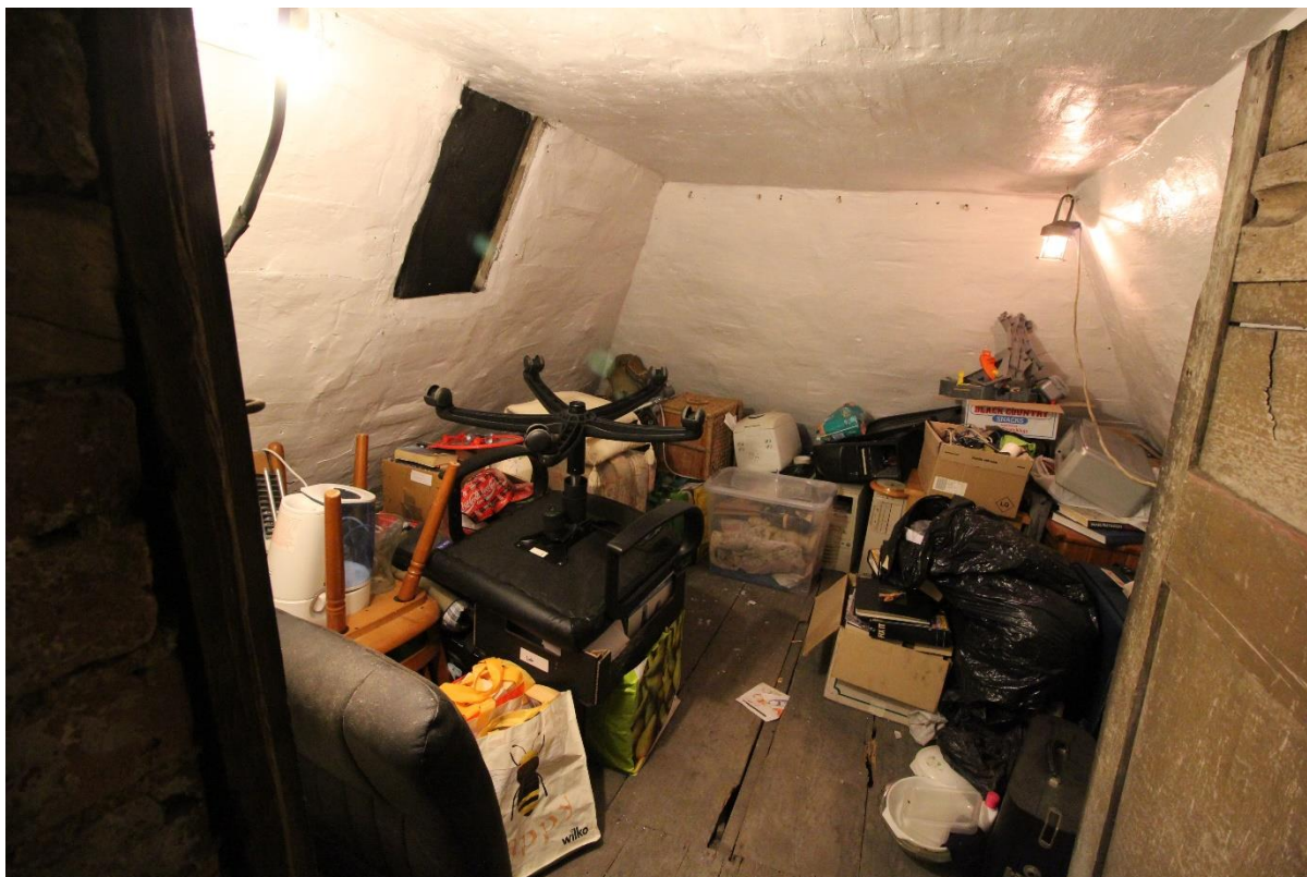
Figure 18 Southern bay attic, note the width of the floorboards, looking south
