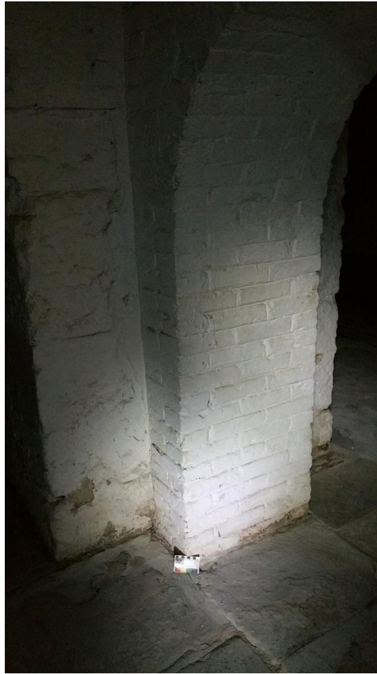
Central Pillar with abutting 'floating' 18th cent brick arches (Location 17)
