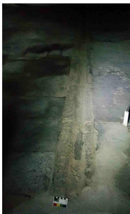
Example of drainage channel in Area B (Location 19)
