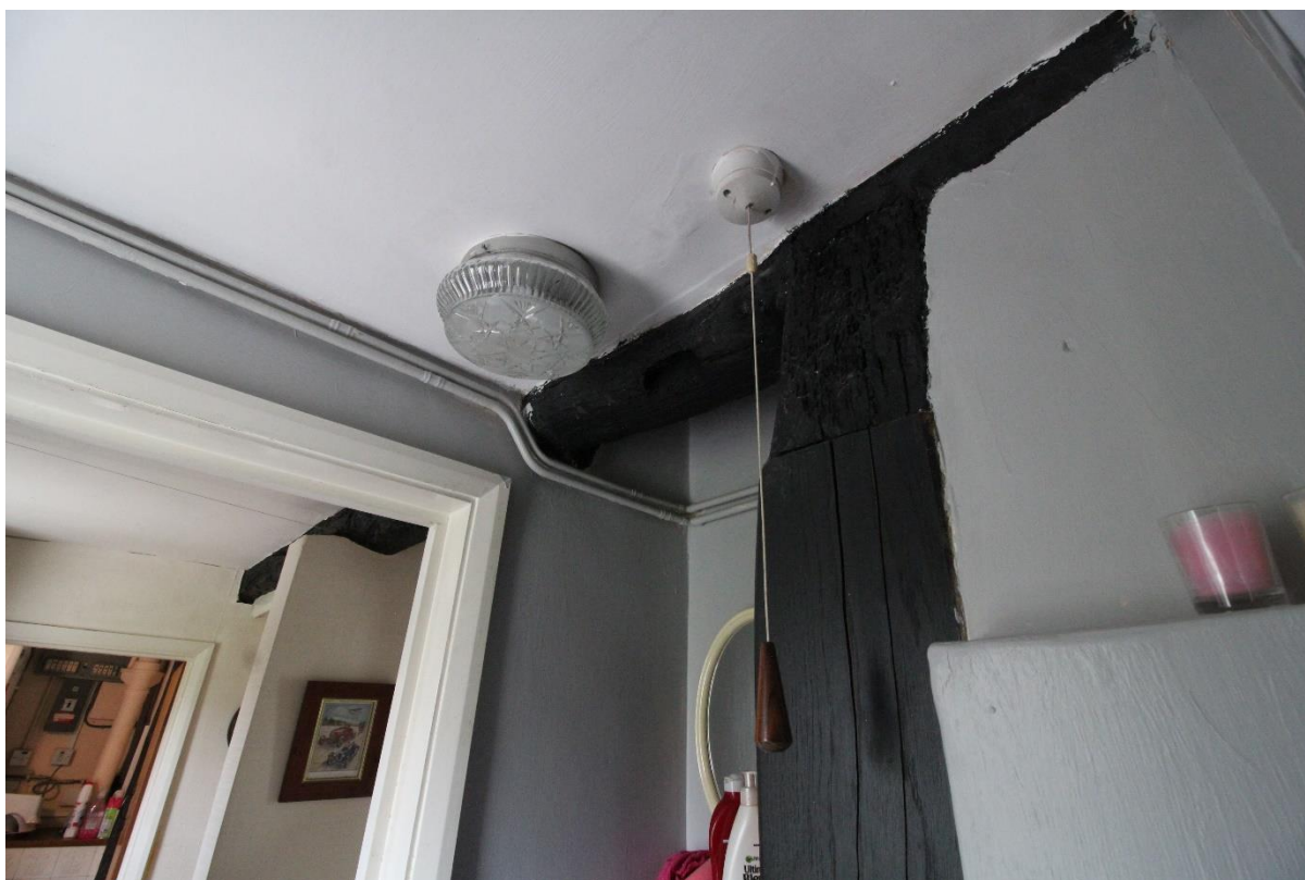
Figure 11 Timber-framing of the former external west elevation, looking north-east
